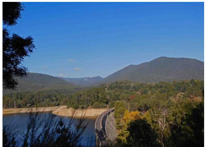
Maroondah Dam. Photo: Heather Ducat
